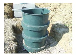
Figure 5. Dosing siphon - external view
