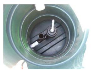
Figure 6. Dosing siphon - internal view
