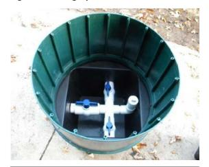
Figure 7. Service box within the manifold line. Ball valves are installed in the manifold to allow isolation of each half of the sandfilter when flushing the distribution network
