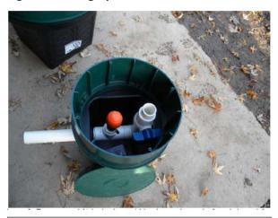
Figure 8. Turn-up and ¾ inch air gap/ bleeder at the end of each lateral for routine maintenance
